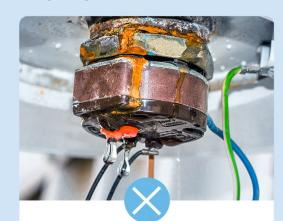
Water or Electric Leakage from tank
