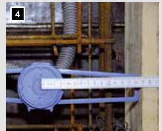
Simply line up the wings simply up to the box centre (15 cm long) on the door frame.
