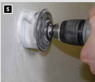
5 You can mill the box hole without re-measuring the mounting location.
