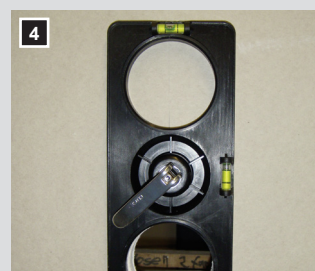
4 Attach the drilling template with the tensioner.
