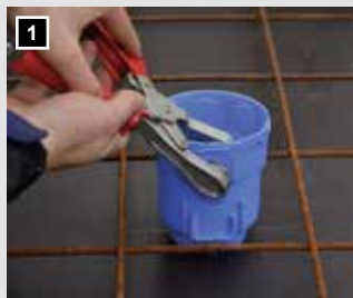
1 Punch out hole with crimping pliers.
