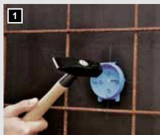
Fix device lid or light outlet cover with nails on the formwork
