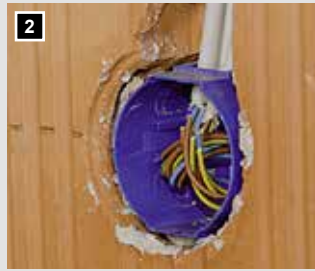
2 Insert the electric cables or pipes.
