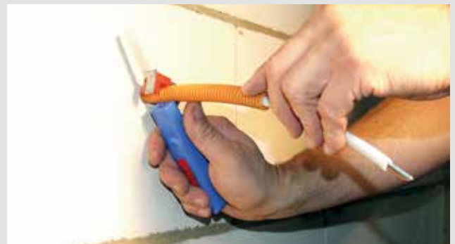
2. Cut off conduit flush with the wall.
