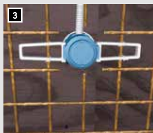
3 Assembly with wings on the steel reinforcement/electronics box.
