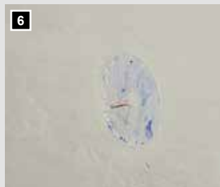
6 The box is found quickly with the plaster pen.
