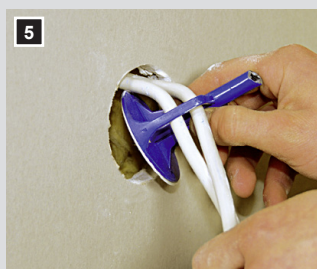
5 Draw pipe brackets and pipes out of the wall.
