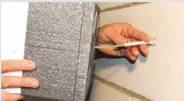
5. Plug the cable into the pre-drilled leadthrough.
