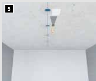
With a hole cutter, the individual opening is drilled out and patched onto the mineral fibre plates.
