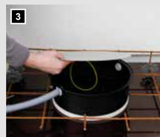
Insert the tubes/cable and secure stable steel plate with cable ties.
