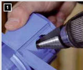
Bore out tube holes.
