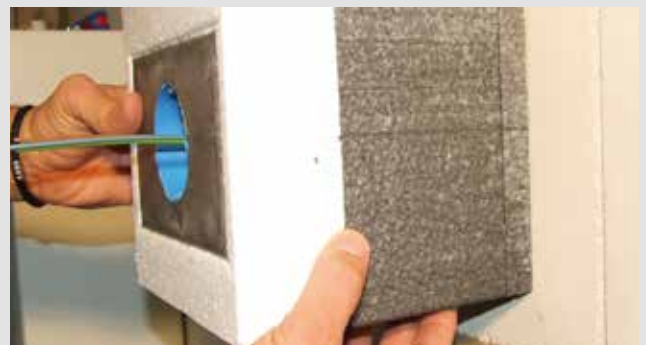
6. Press element - sets after approx. 2 min.
