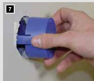
7 Insert the upper part of the box and push until flush.
