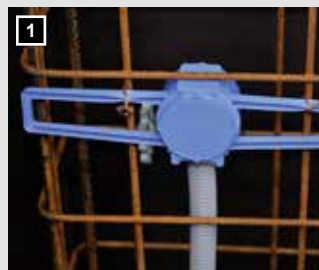
Insert tube and simply tie on the steel reinforcement.
