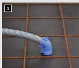
4 Stick onto the lower part. Absolutely secure strain relief!
