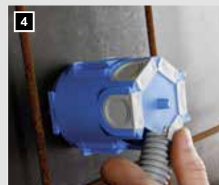
Insert and close tube with quick-fix slide.
