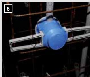
5 Assembly as electronics large box with wings.
