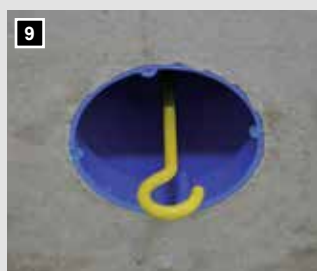
Mounting a ceiling box with terminal box and support for ceiling hook.
