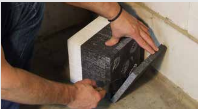
1. Adjust the insulation thickness, i.e. disconnect 20 mm insulation plates.
