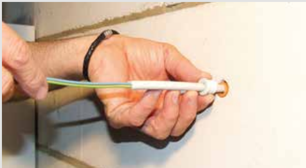
3. Wind-proof lock conduit with sealing plugs (included in the delivery).
