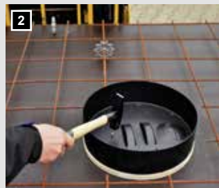
In site concrete, nail on formwork or glue in the precast factory on sound table.
