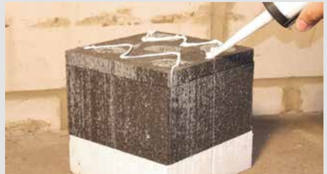
4. Apply TIE hybrid adhesive in thin beads (5-6 mm).
