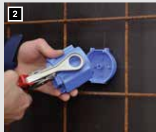
Punch out pipe or cable inlet using the crimping pliers.
