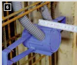
The mounting of the inverted wing concrete box also allows a concrete cover up to 60 mm.
