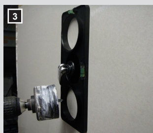
3 Then drill through the existing hole inserts.
