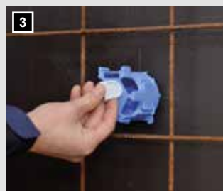
Close unused openings with slide.
