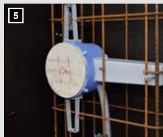
Assembly with wings and transformer tunnel.
