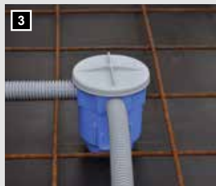
3 Assembly as ceiling large box.
