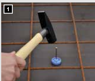
1 Nail lower part on the formwork.
