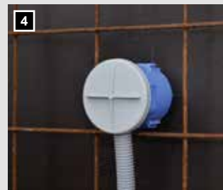
4 Wall mounting as electronics large box.
