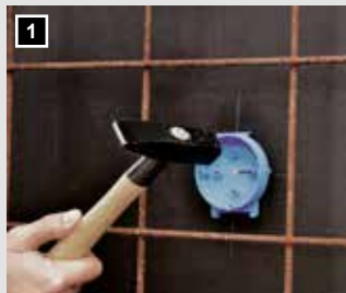
Attach device lid with nails on the formwork
