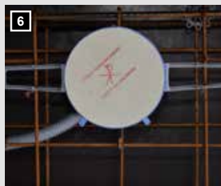
XL 170 without transformer tunnel, installation with wings.
