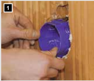
1 Set the box lower part flush with the brickwork.
