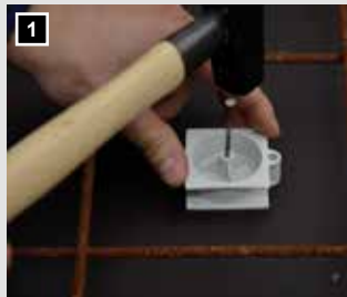
Nail base on the formwork.
