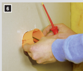
6 Without a long time searching for cables, you can install the cavity wall box.
