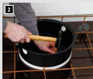
In site concrete, nail on formwork, glue in the precast factory on sound table.
