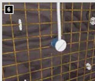
6 Insert tubes and use e.g. as electronics box or large terminal box.
