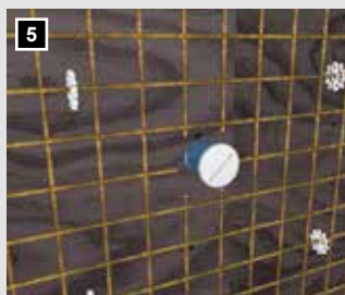
5 Universal large box can be mounted in the wall with nails.
