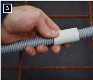
Secure strain relief - done!
