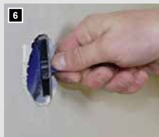
6 Gently take out the milled-through drill press.
