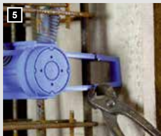
Simply tie onto the steel reinforcement. Concrete cover up to 40 mm.
