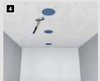
4 Knock out opening with a hammer.
