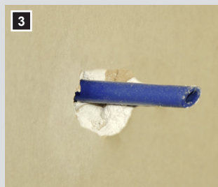
3 The dry wall builder knocks out a hole with a hammer and lets the central spike get through, this serves as a centre for the drill bit.
