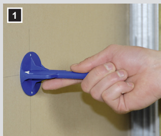
1 Glue the pipe bracket on the back of the first cladding.
